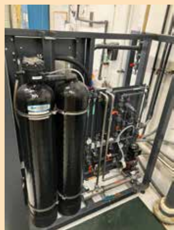
New Hypochlorite Generation System at DMTP
