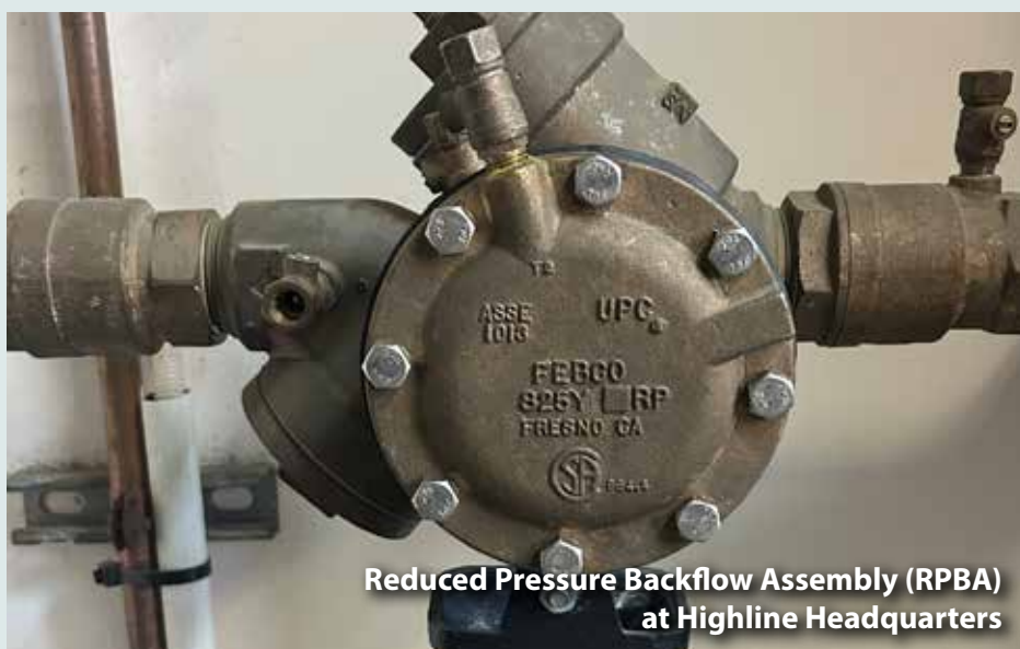
Backflow Assembly Being Tested
