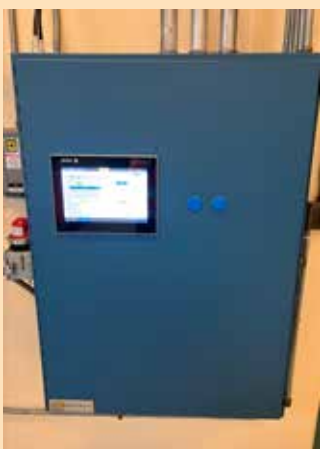
New Telemetry System at PS6
