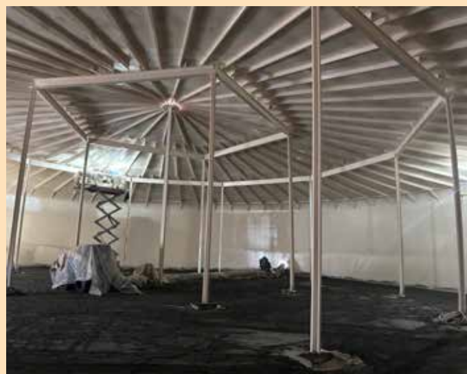
Interior of 2.5 MG Reservoir during rehabilitation
