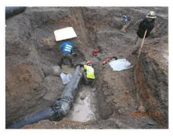
This project replaced approximately 7,700 LF of existing AC water mains with new, ductile iron pipe, in addition to new services, hydrants, services and appurtenances. Staff selected the project locations due to recent water main breaks, proximity to sensitive environmental areas and in anticipation of future city overlay projects.
