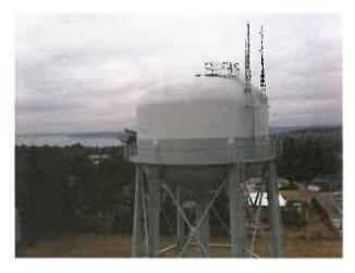
Project 16-3 includes the construction of a new, 4.5 MG 490 Zone reservoir to replace the existing 5.0 MG reservoir; however, the new location will conflict with the existing 0.25 MG elevated tank. The project includes the demolition of both tanks. The elevated tank will be replaced by the proposed pump station identified as Project 16-6.
