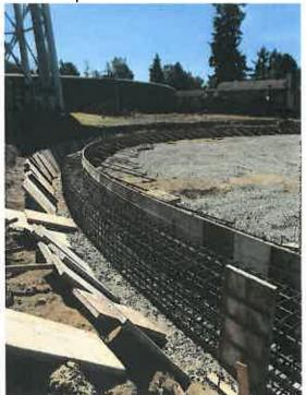
Project 16-3 includes the construction of a new, 4.5 MG 490 Zone reservoir to replace the existing 5.0 MG reservoir; however, the new location conflicted with the existing 0.25 MG elevated tank. The project includes the demolition of both tanks. The elevated tank will be replaced by the proposed pump station identified as Project 16-6.
