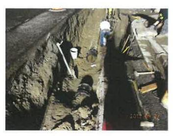
A second break occurred on August 13, 2018 at 5 240th St and 9th Place S. An existing service line broke at the water main causing the pipe to rupture. The break caused significant damage to one existing home. During the repair, the 4-inch AC water main was observed to be soft and in poor condition causing the District concern over potential future ruptures.
