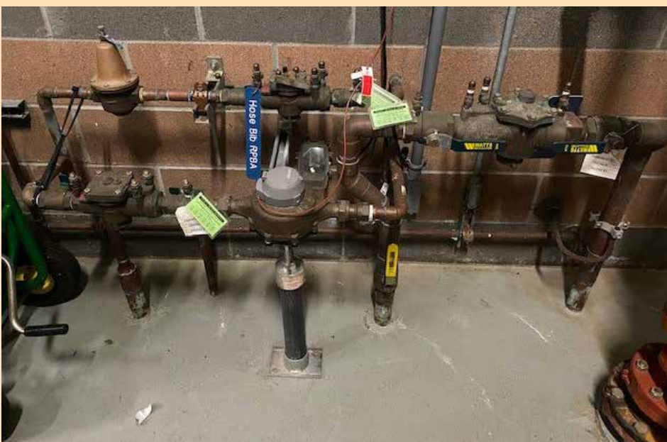
Backflow Assembly Being Tested
