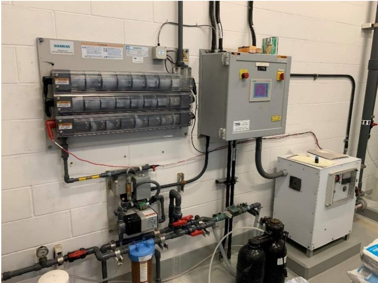
The District operates a Wallace & Tiernan onsite hypochlorite generation system at the McMicken Treatment Plant. The unit uses salt and electricity to create a weak solution of sodium hypochlorite (bleach) used for water disinfection at the treatment plant. The system has been in operation for 10 years and is nearing the end of its useful life.
